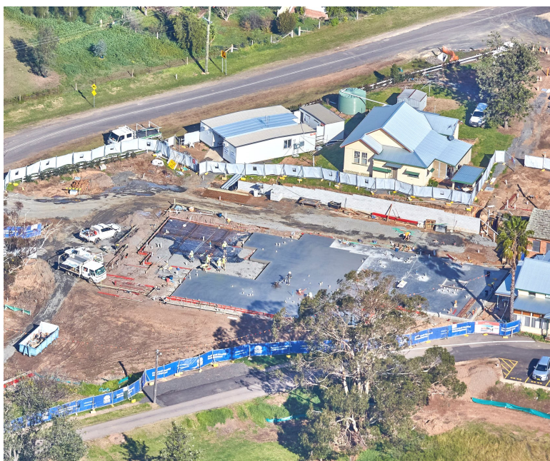
Aerial photo taken in late May, showing the concrete ground slab after the second day in the pouring process
