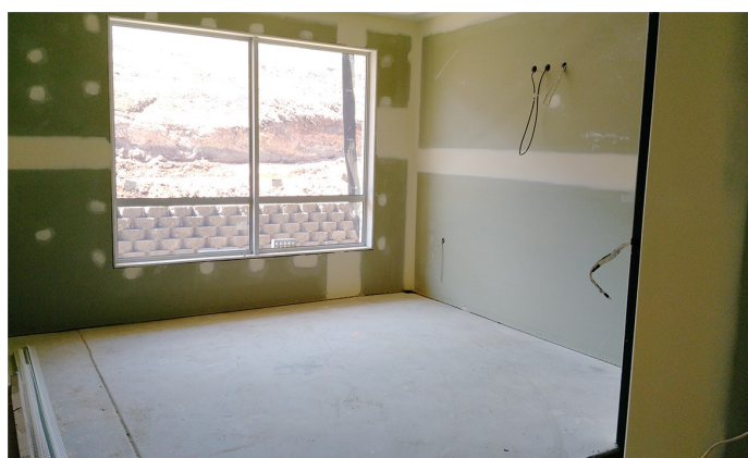
Internal wall sheeting is completed in the emergency department.
