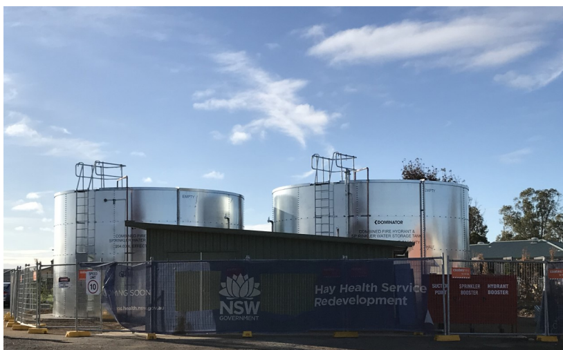
Below: The two new hydrant and sprinkler tanks have been installed as part of the fire protection system.
