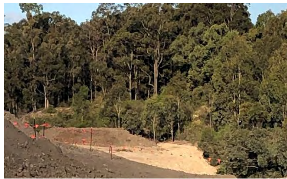
Figure 5 Separation of topsoil and mulch stockpile
