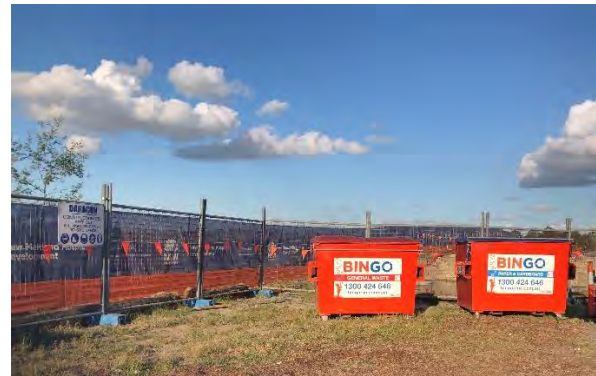
Figure 2 Waste bins and site fencing
