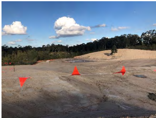
Figure 1 Sediment basin and well compacted earth works
