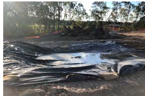
Figure 4 Concrete washout and separation of timber for mulching in background
