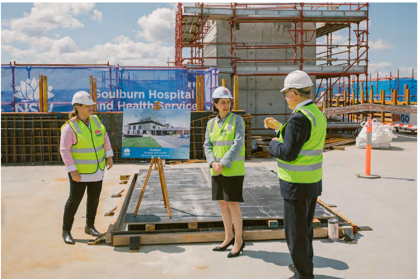
Topping Out at Goulburn Hospital and Health Service Redevelopment. (29 September 2020) Left to right: Member for Goulburn Wendy Tuckerman, Premier Gladys Berejiklian and Health Minister Brad Hazzard
