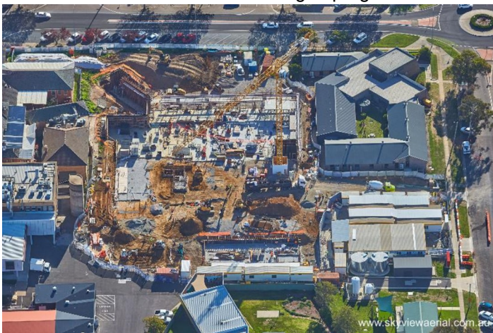
Aerial images of Goulburn Hospital and Health Service Redevelopment April 2020
