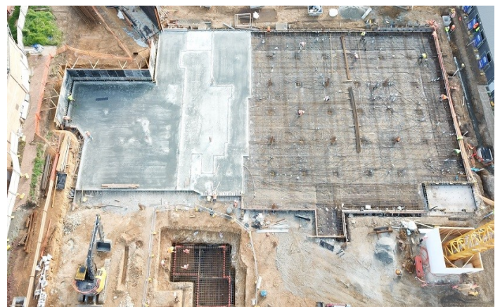
Concrete slab pour at Goulburn Hospital and Health Service Redevelopment site
