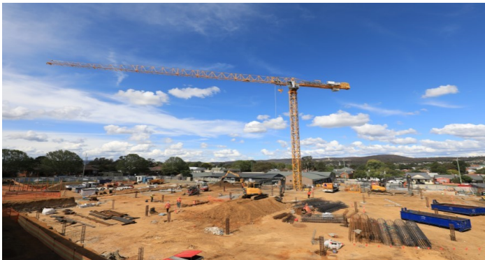
Tower crane arrives at Goulburn Hospital and Health Service
