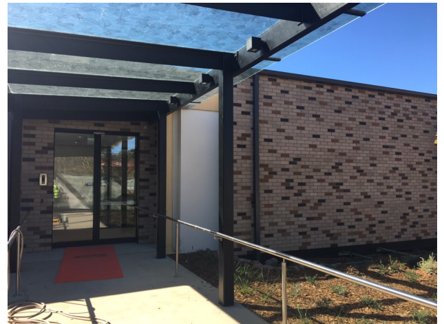
New main entrance to Cooma Hospital.
