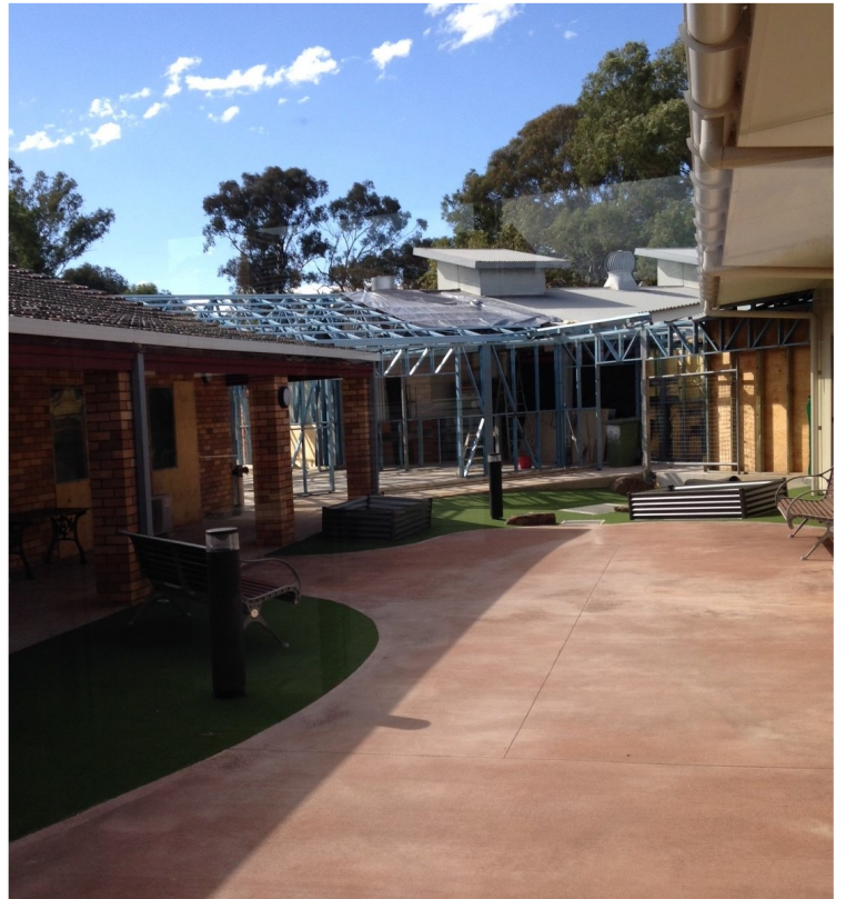
Photo above: The new “Magnolia House” Residential Aged Care wing is nearing completion, as seen from the internal courtyard (not yet complete) attached to “Rosella Place”.
