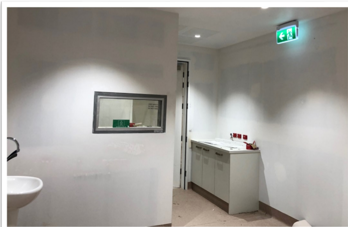
The X-ray room, taken from where the X-ray machine will sit, looking back towards the room's entrance.
