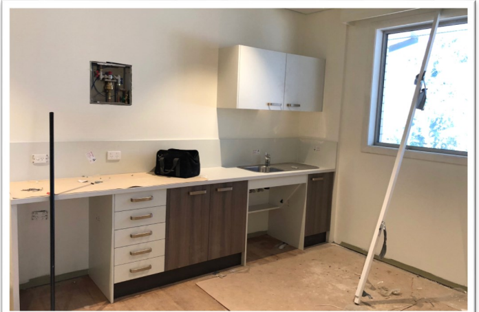
The kitchen facilities in the new meeting room, being built as part of Stage 2.
