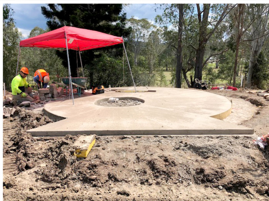
The formwork for the centerpiece of the Aboriginal Garden.
