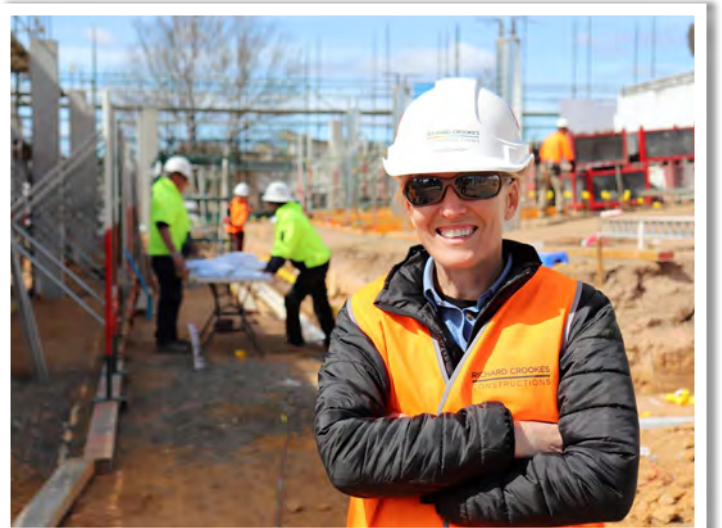
Richard Crookes Constructions forges ahead on the Braidwood MPS Redevelopment project.
