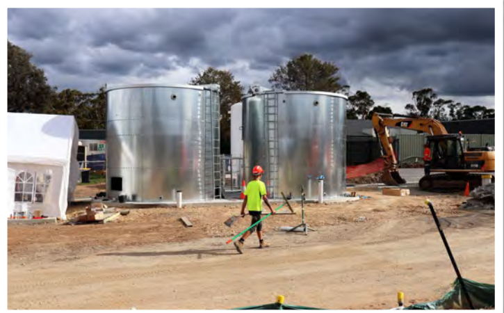
The new water tanks at Goulburn.
