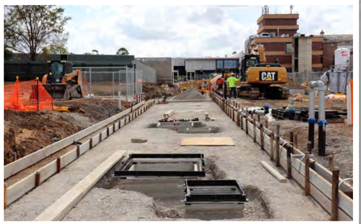
The new main services trench.
