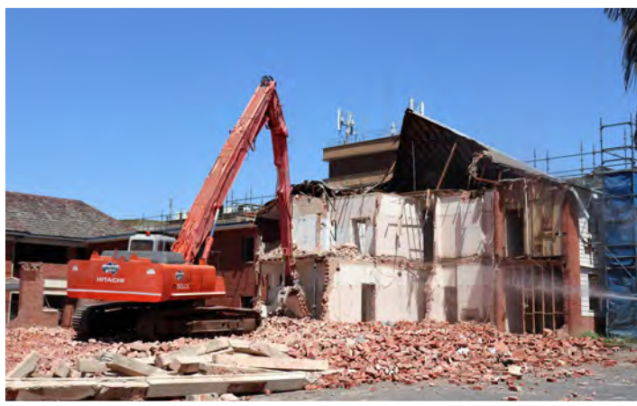
Clearing the way for the new four storey clinical services building.
