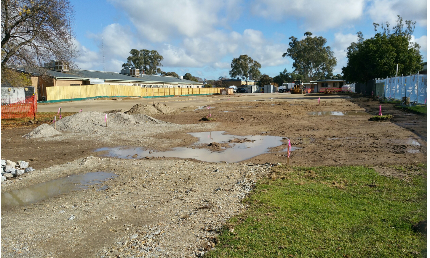
The demolition of Eliza House has made way for the new Barham MPS.
