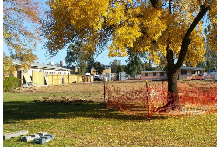
The Barham MPS is due for completion in 2020.
