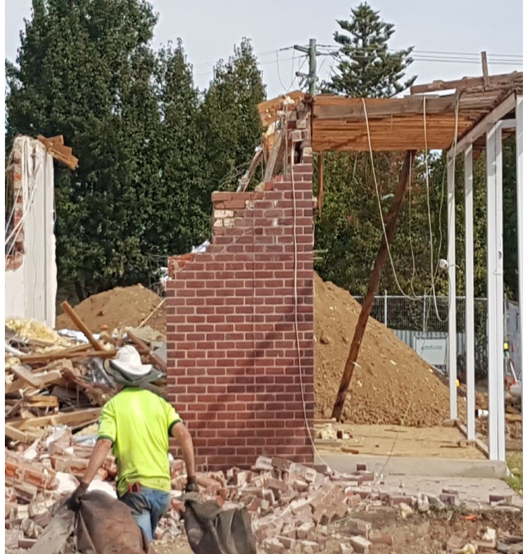
The last wall standing on the Culcairn site.
