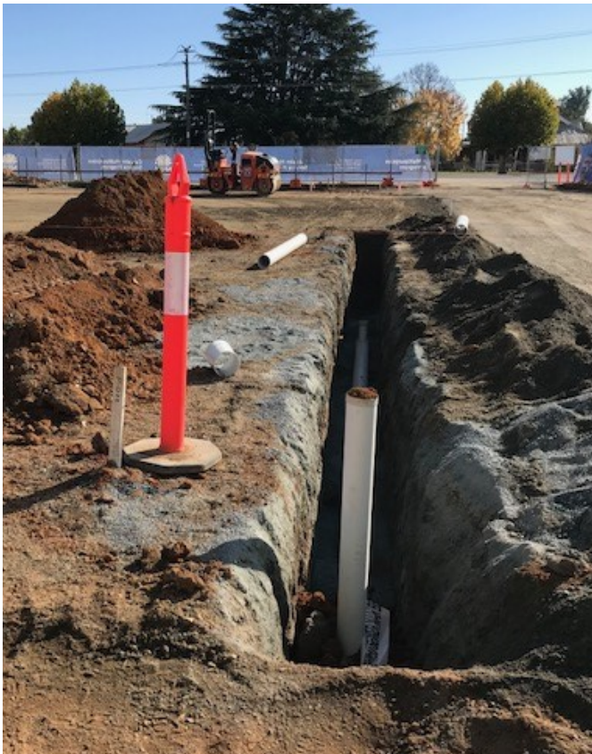
The footings for the Culcairn MPS are being installed.
