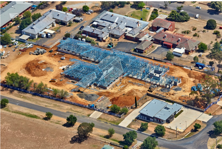
Above: A view of the Health Service under construction in late 2019
