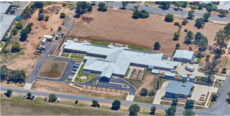
Above: A view of the Health Service nearing completion in late January 2021
