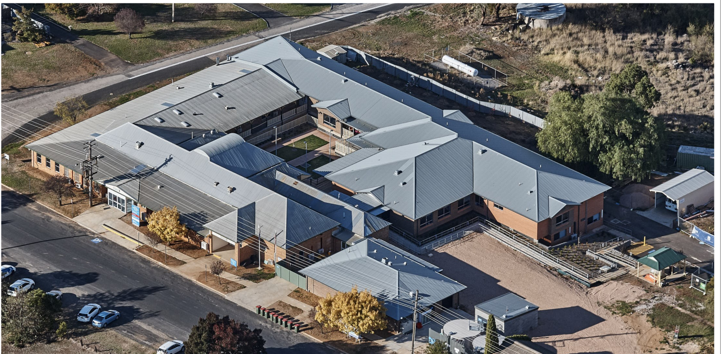
Photo: Aerial image of the Molong MPS taken in late April 2018, showing the work completed on the new 'Support Services' building (bottom of photo) and front entry, as well as the new RAC section taking up the entire eastern side of the MPS.
